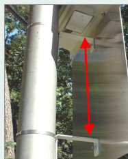
Installed extender brackets
