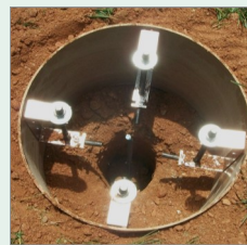
Installed concrete form with anchor bolts & rebar
