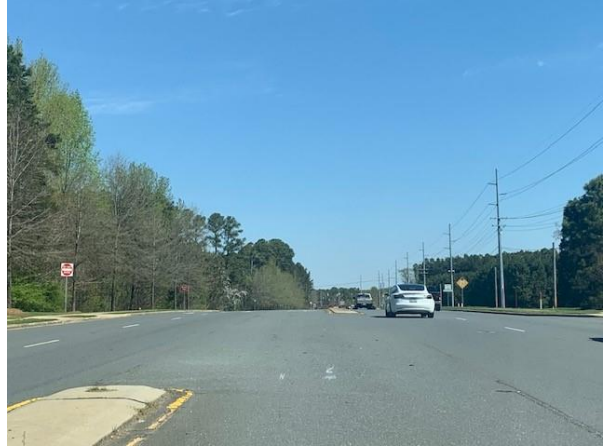
Providence Road facing north at Old Mill Road/Access “A”
