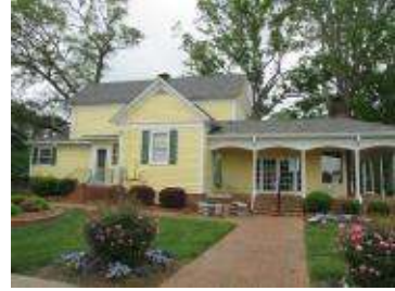
Painting to the specified surfaces of the back of Town Hall.
